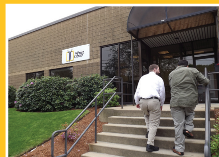
The Price Center's new location at 77 Rowe Street.
