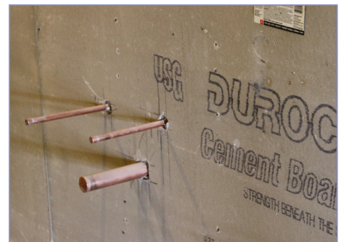
Construction is in progress at The Price Center’s new home at 25-27 Christina Street in Newton.
